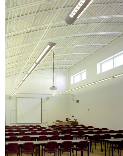
High window placement and even distribution reduces glare and provides a more even distribution of light in the space.
