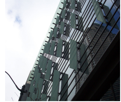
Vertical shading on the east and west facades handle low sun angles in the morning and evening.
