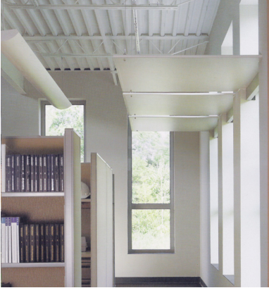
Interior lightshelves stop direct solar penetration onto work surfaces and also increase daylight penetration.
