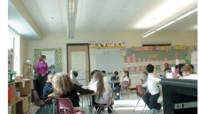
Light fixtures and circuiting parallel to the window walls allows dimming systems to better compliment the natural daylight.
