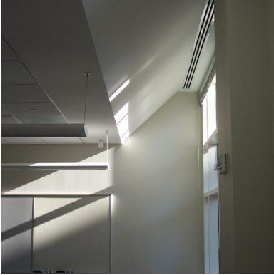
Sloped ceilings and windows placed as close as possible to the ceiling increases daylight penetration.
