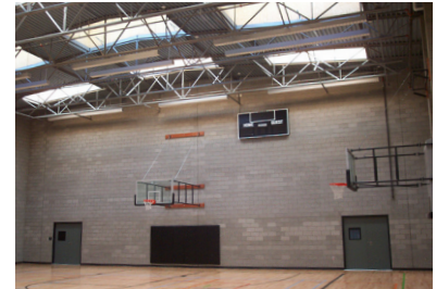
Evenly distributed toplighting provides ample lighting for large spaces.
