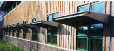
The sun travels in an arc through the sky, therefore, shading devices and lightshelves should extend past the window for full shading.
